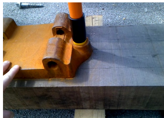
1. INSERT AND SCREW TO FULL DEPTH.
