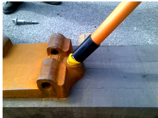
2. LEAN WITH THE BAR TO MOVE THE FERRULE.
