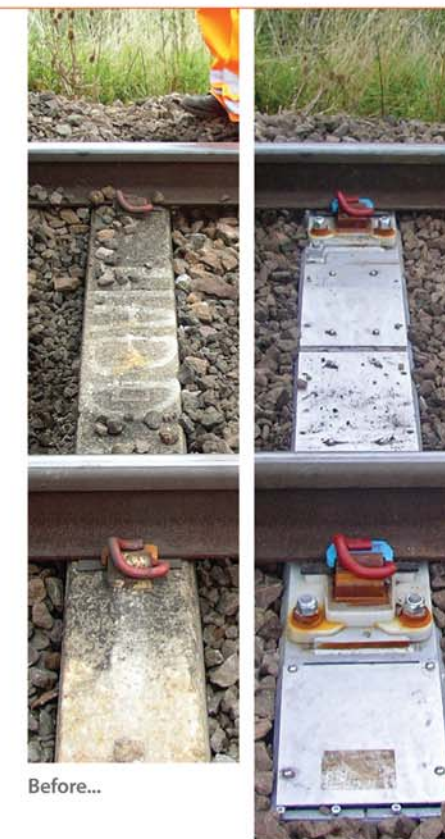
...and after the installation of a Tenconi hollow sleeper.
